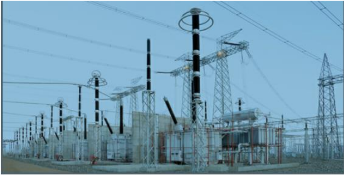
CPRI Testing Site Visited by Students
