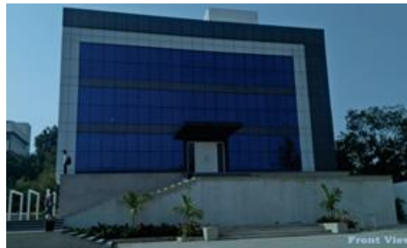
R&E Hub Front View
