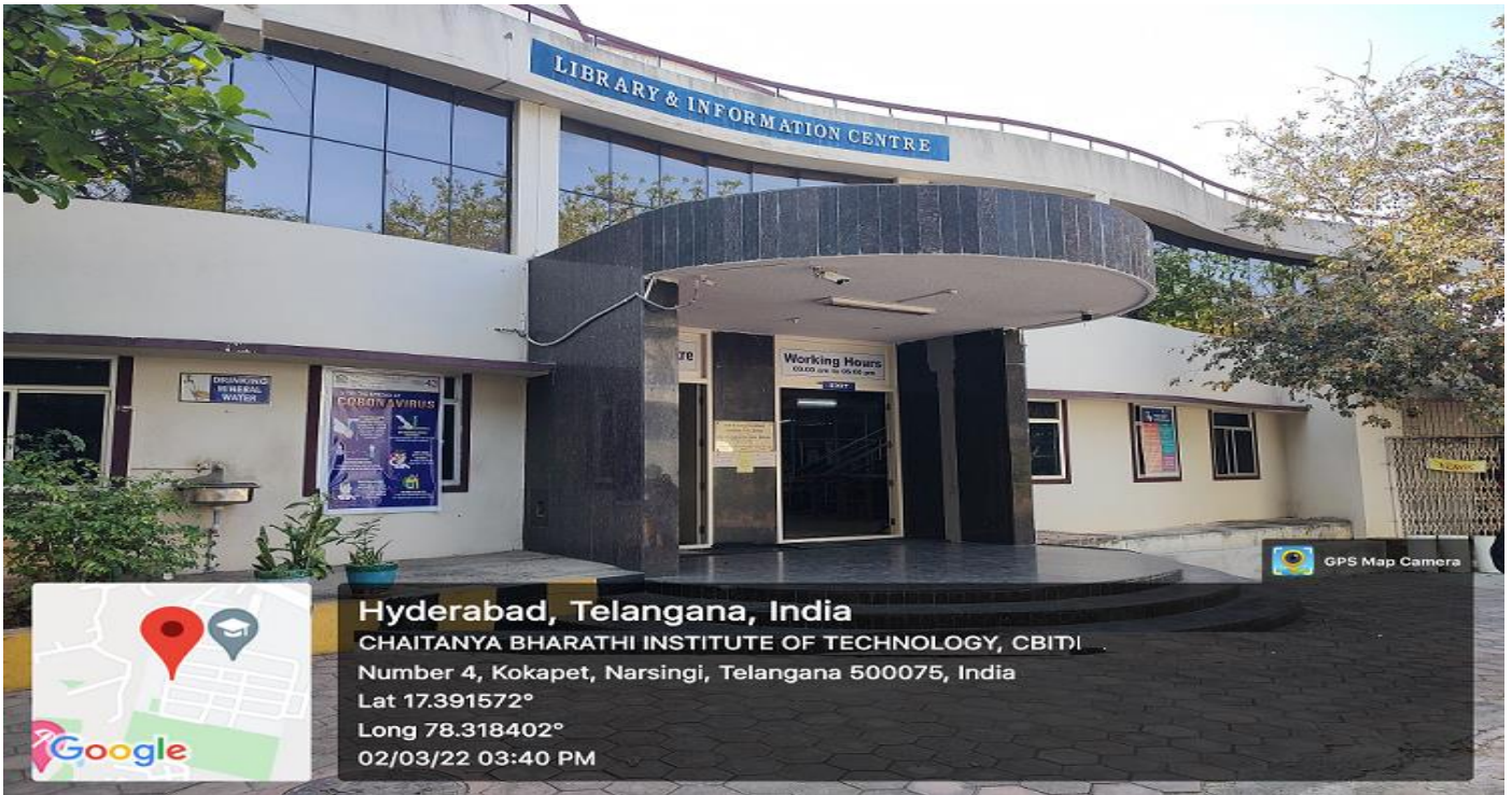
LIBRARY FRONT VIEW
