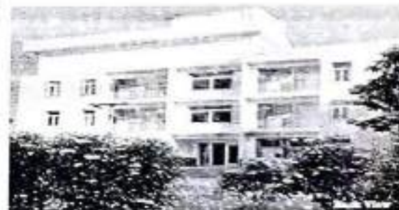
R&E Hub Back View
