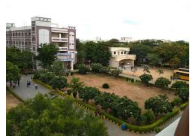
EEE department Front View
