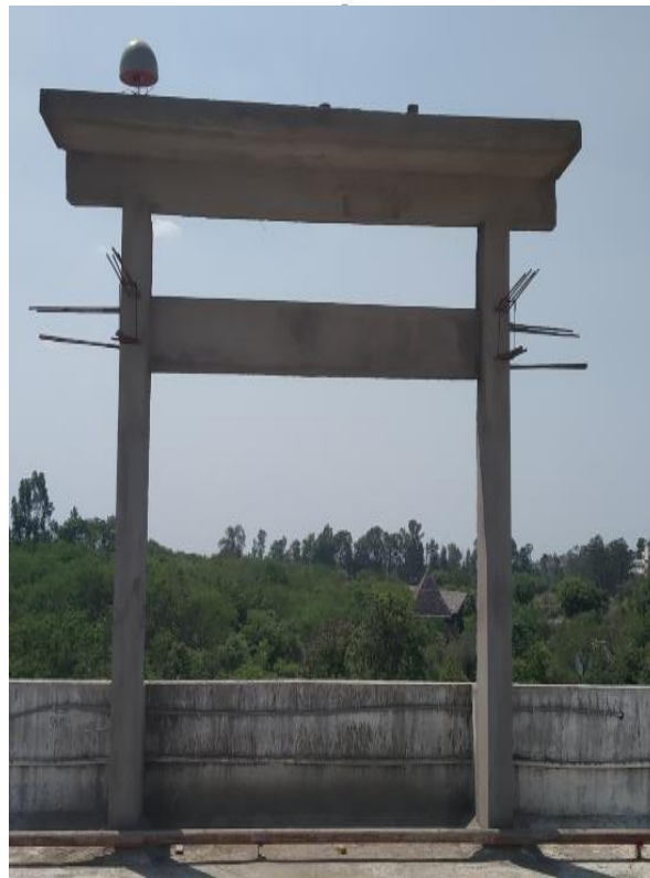
Fig. 3. PoLaRx5S Receiver Antenna mounted at rooftop of R&E Hub
