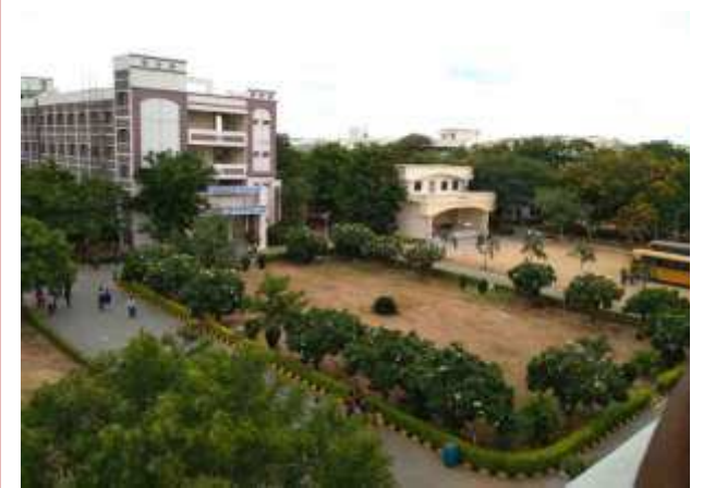
EEE department Front View
